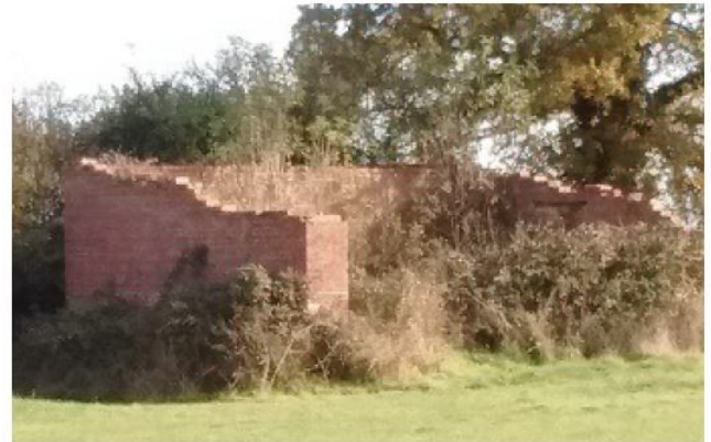
Remains of a blast wall which would have surrounded the transmitter hut—this one survives at Templecombe.
